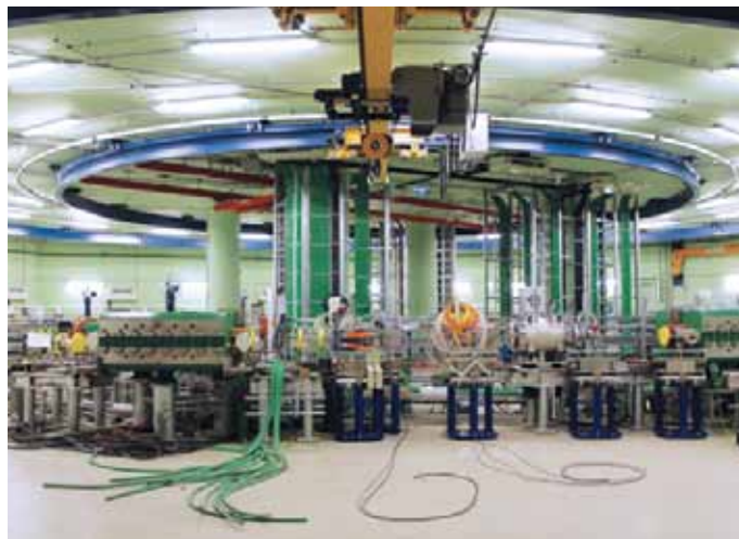
Installation of the synchrotron at MedAustron
